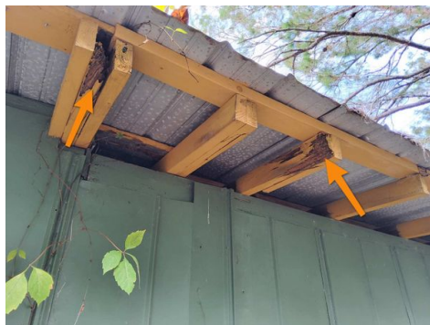
Rear of the bathroom
