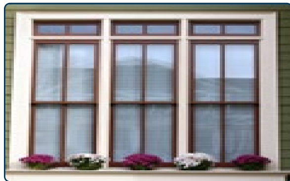
Figure 138: Example of appropriate fiberglass windows.
