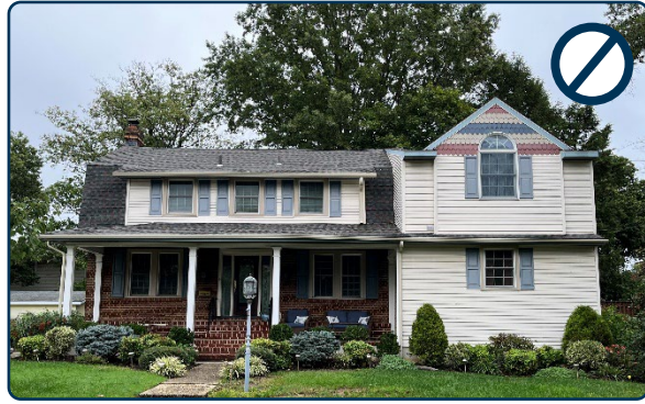
Figure 110: Inappropriate new addition with an incompatible scale, height, and use of materials.
