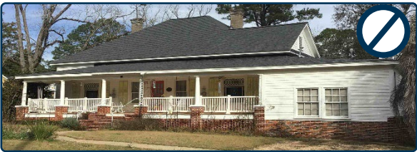
Figure 98: Inappropriate side addition that is not setback.
