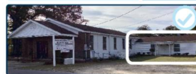
Figure 97: Many religious properties have constructed rear additions as programming expanded or as the congregation grew.
