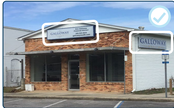
Figure 55: Appropriate signage on a gable roof commercial building.
