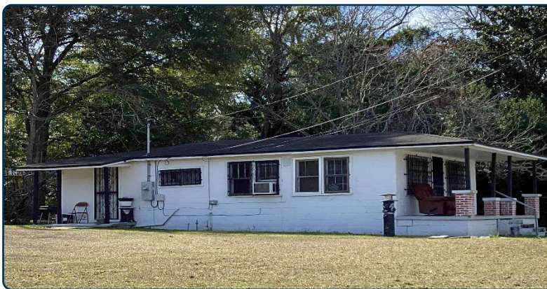
Figure 106: Many residential and commercial buildings were constructed with concrete block. New construction utilizing concrete block would be appropriate.
