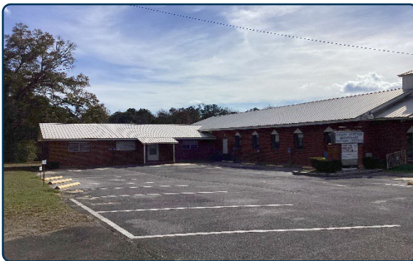
Figure 28: Maintained parking lot associated with a religious building in the district.
