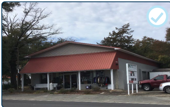
Figure 91: Many gable roof commercial buildings are clad in metal.
