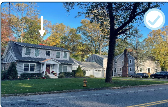
Figure 115: Appropriate new construction with compatible massing, alignment, scale, rhythm, and materials.
