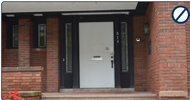
Figure 108: Example of an inappropriate front door that is too simple and is not compatible with a residence.
