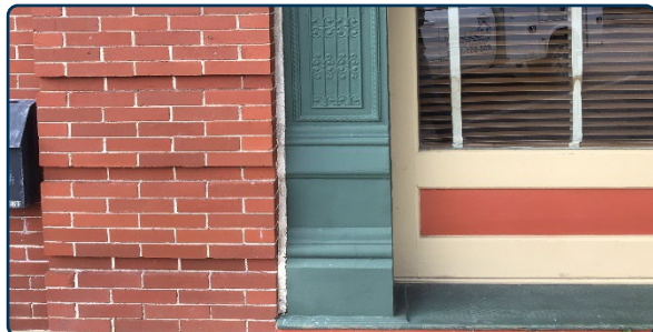
Figure 119: Cast iron pilaster and wood bulkhead that should continue to be painted for protection.
