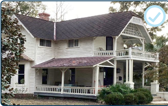
Figure 86: Many historic residences feature scalloped asphalt shingles.
