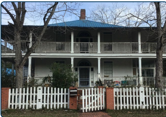
Figure 60: Historic residence that features wood windows, siding, porch elements, and fencing.
