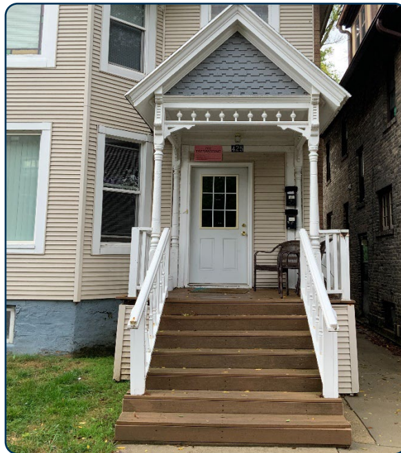
Figure 141: Porch flooring and steps replaced with compatible substitute material similar in visual qualities.
