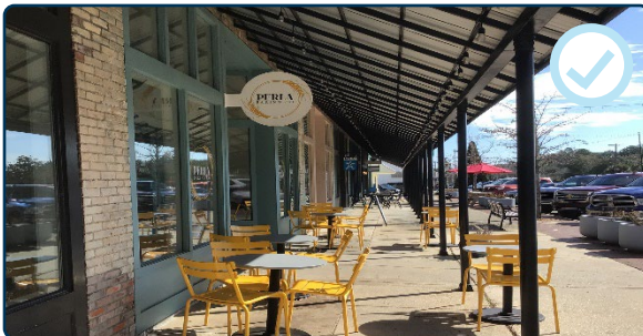
Figure 94: Appropriate porch addition on the front a commercial block.
