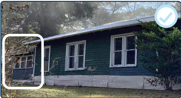
Figure 99: Appropriate rear addition on a historic residence.
