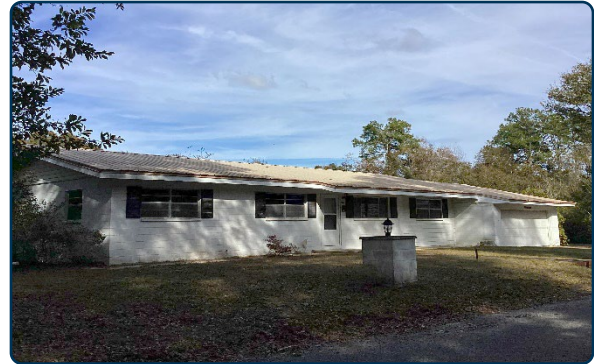
Figure 16: Example of Ranch building type in the Dorsey Avenue Historic District.
