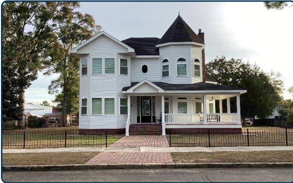
Figure 40: Residence without a front driveway. The addition of a new driveway accessible through the front yard would be inappropriate.
