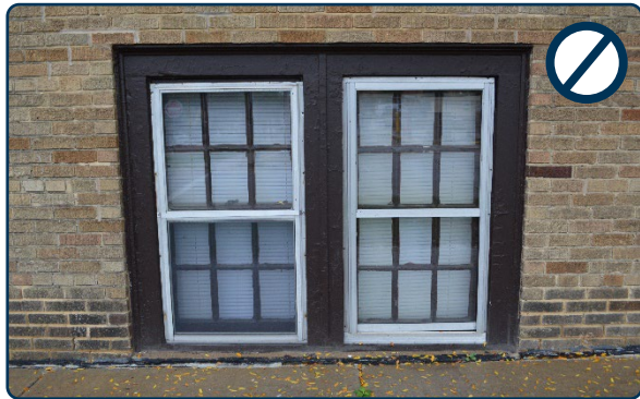
Figure 69: Inappropriate storm windows that obscure the original windows.
