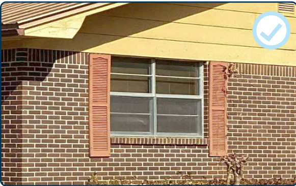
Figure 68: Many residences feature decorative shutters around the windows.
