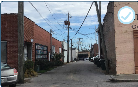
Figure 105: Appropriate location of general utilities on side and rear façades within an alley in the commercial district.
