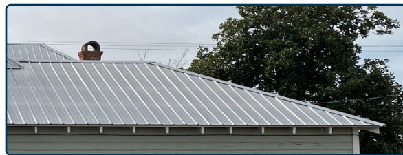
Figure 147: 3-V crimp metal roofing.
