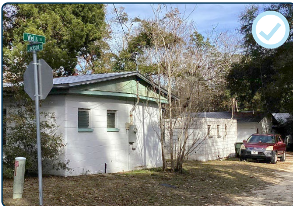
Figure 55: Several masonry vernacular concrete block historic residences are located within the district, with varying conditions.
