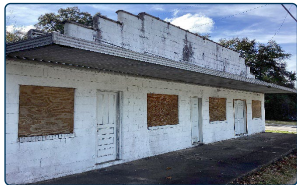
Figure 17: Example of a One-Part Commercial Block building type in the Dorsey Avenue Historic District.
