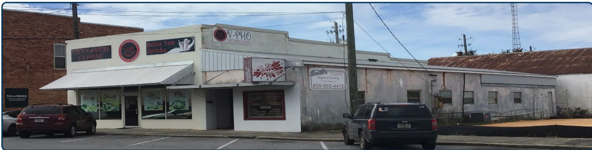
Figure 90: Masonry vernacular flat roofs also commonly feature stepped parapets.
