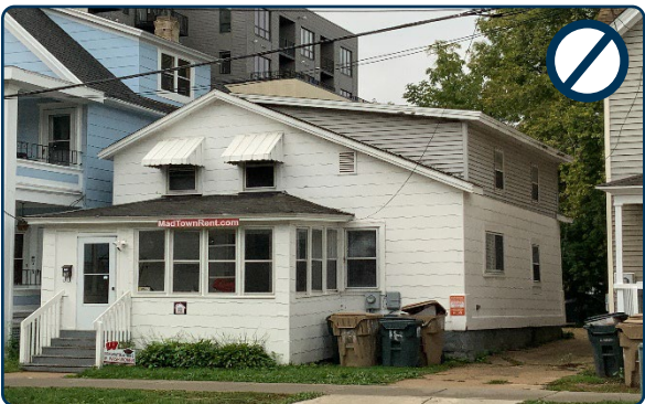
Figure 74: Inappropriate roof dormer addition on historic building.
