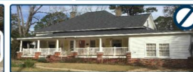
Figure 98: Inappropriate side addition that is not setback.
