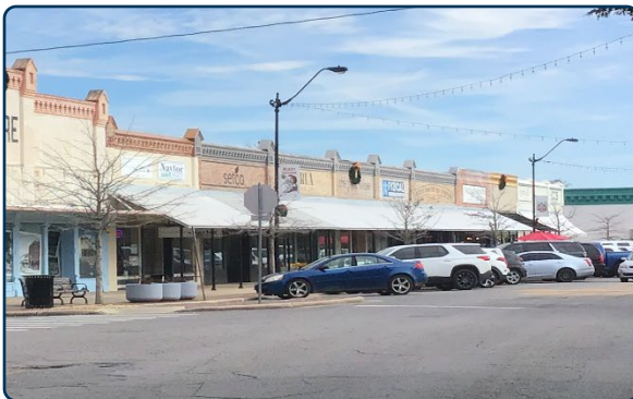
Figure 37: Angle parking along Main Street, typical throughout the commercial area.
