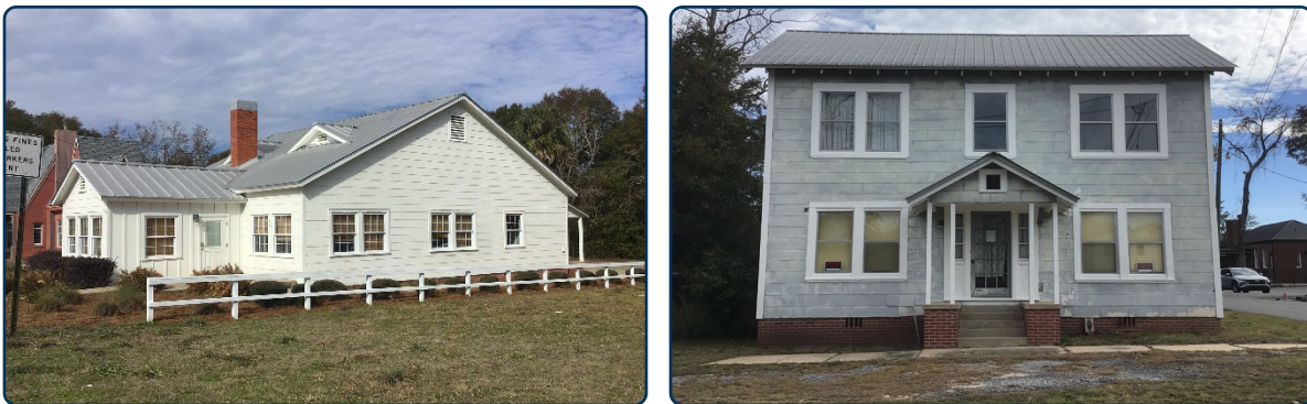
Figure 22: Examples of a frame vernacular commercial properties in DeFuniak Springs.
