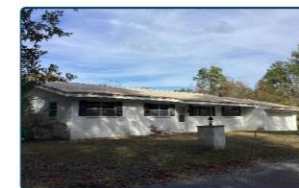
Figure 16: Example of Ranch building type in the Dorsey Avenue Historic District.
