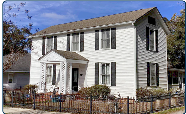
Figure 15: Example of a residential Single Pile building type in DeFuniak Springs.
