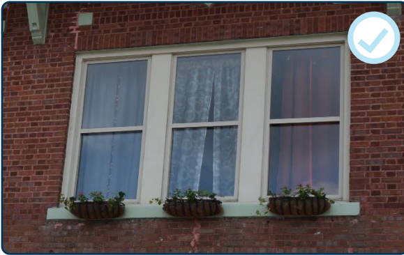
Figure 83: Appropriately preserved wood window types.
