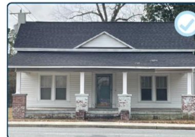
Figure 64: Example of appropriate replacement siding on a historic residential building.
