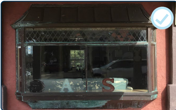
Figure 85: Maintained character-defining window on commercial property.
