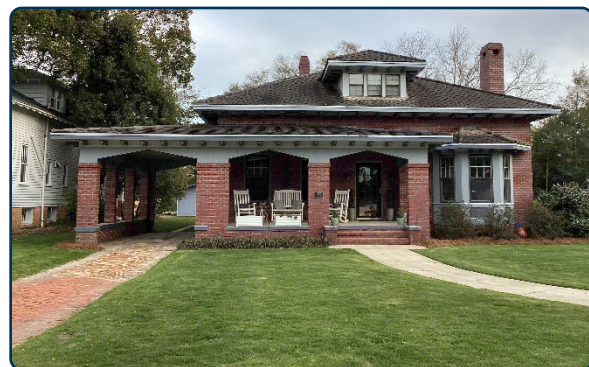
Figure 39: An appropriate brick paver driveway and paved concrete walkway.
