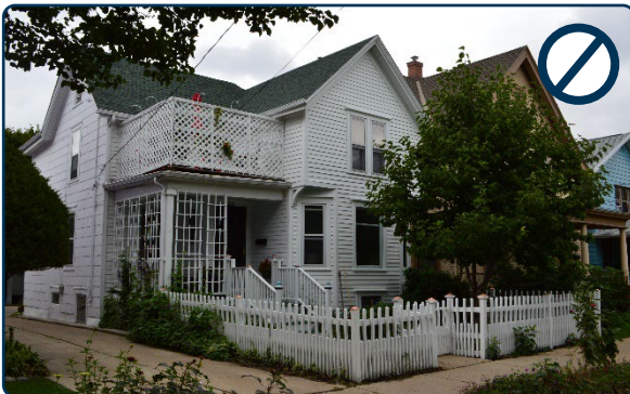
Figure 45: Inappropriate variety of fencing surrounding a historic residence.
