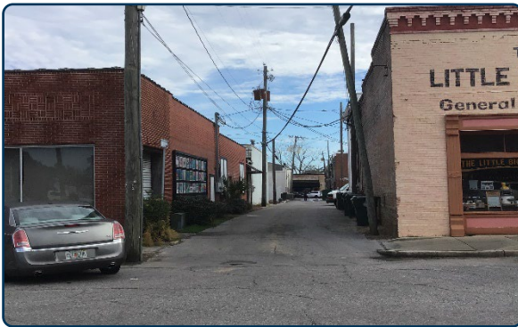
Figure 35: Example of a paved alley within the commercial core.
