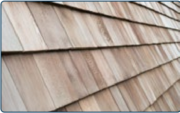
Figure 129: Unpainted wood shingles.
