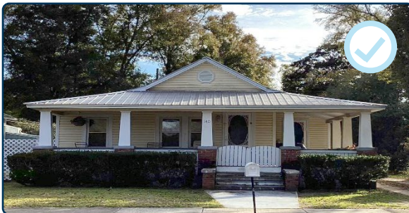
Figure 91: The porches of many Craftsman style residences in the district feature columns on piers.
