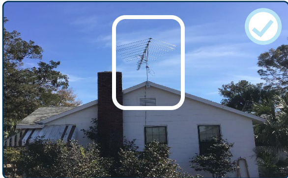
Figure 93: Appropriate location of an antenna on the side elevation of a historic residence.
