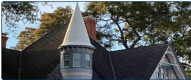
Figure 72: This historic residence features a variety of character-defining details that define its Queen Anne architectural style. The removal of any would damage the integrity of the residence.
