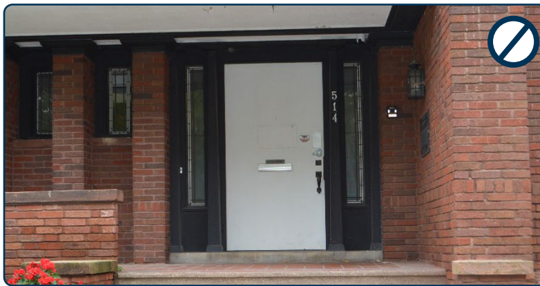
Figure 120: Example of an inappropriate front door that is too utilitarian and is not compatible with the rest of the building.
