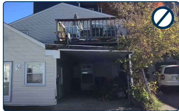
Figure 94: Inappropriate deck addition to the front façade of a residence.
