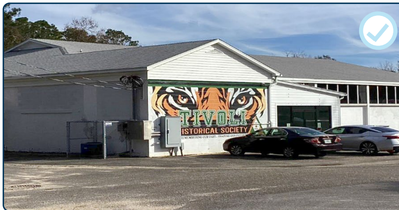
Figure 40: Example of appropriate mural within the historic district.
