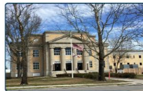
Figure 23: Examples of historic Neo-Classical Revival style institutional buildings in DeFuniak Springs.
