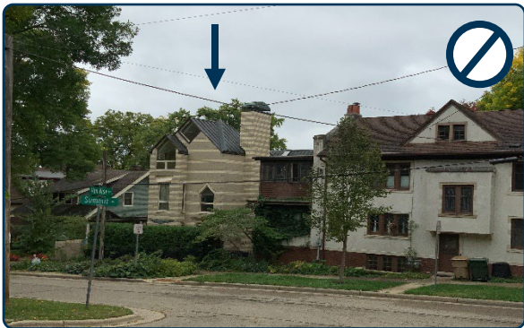
Figure 104: Inappropriate new construction with incompatible massing, materials, scale, height, and rhythm.
