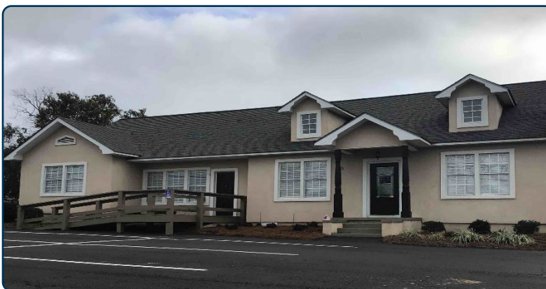
Figure 122: New construction commercial building with an appropriate ramp.
