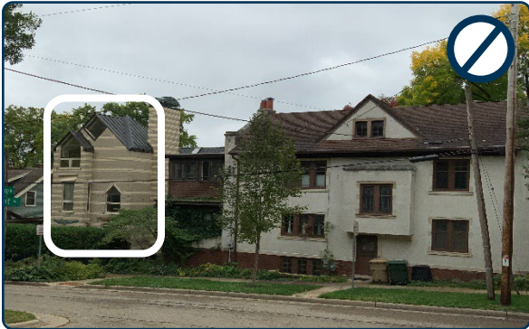
Figure 109: Inappropriate new window shapes on a new residential construction.
