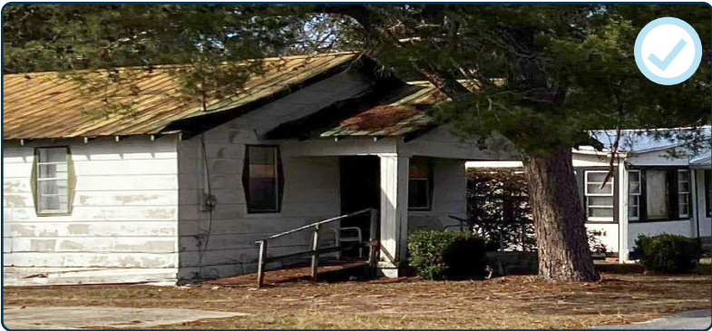
Figure 46: Appropriate wooden ramp on a residential front
