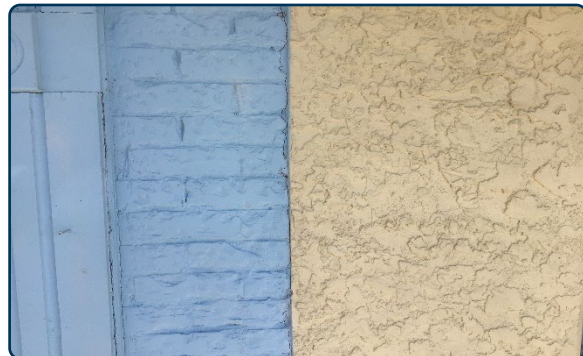
Figure 73: Example of textured stucco applied to masonry within the commercial district.
