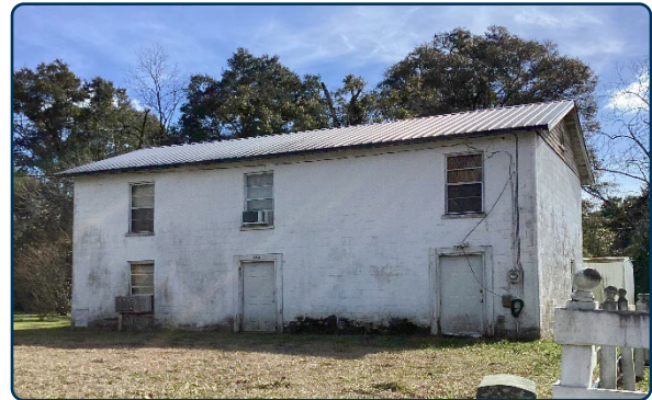
Figure 12: Example of a residential Single Pile building type in DeFuniak Springs.
