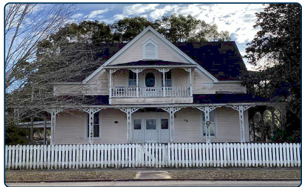
Figure 27: Above are examples of Folk Victorian style buildings in the DeFuniak Springs Historic District.
