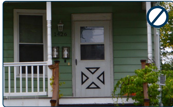
Figure 77: Inappropriate storm door that obscures the original door.
