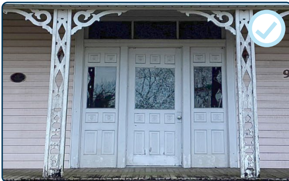
Figure 74: Appropriately preserved historic wood door.
