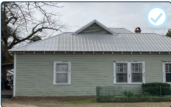
Figure 73: Appropriate metal replacement roof on a historic residence.
