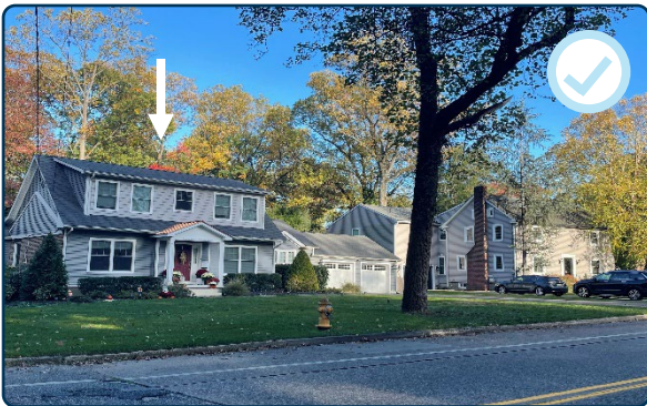
Figure 103: Appropriate new construction with compatible massing, alignment, scale, rhythm, and materials.
