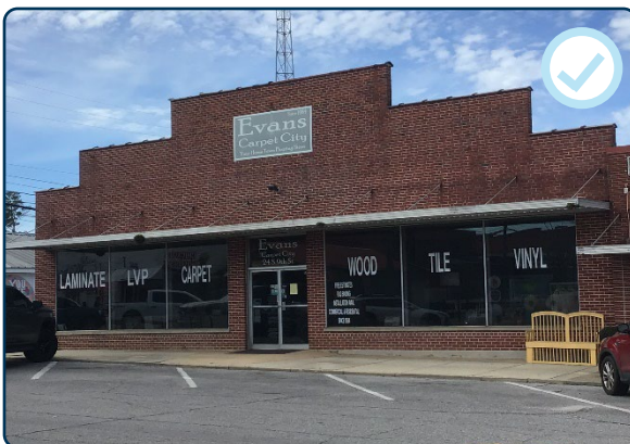
Figure 71: Appropriately maintained historic brick masonry commercial property.
