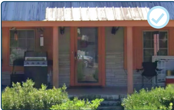
Figure 63: Appropriate storm door that is compatible to the historic residence.
