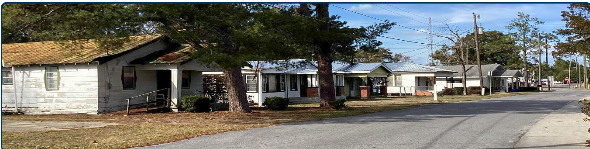
Figure 72: Most roof shapes in the district are gable or hip clad in metal or shingle cladding.
