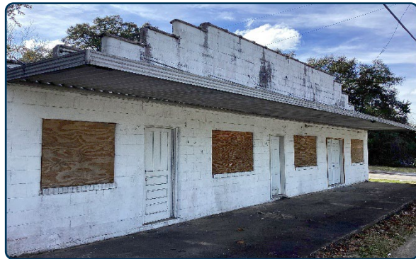
Figure 82: Appropriate metal awning over a commercial storefront entrance.
