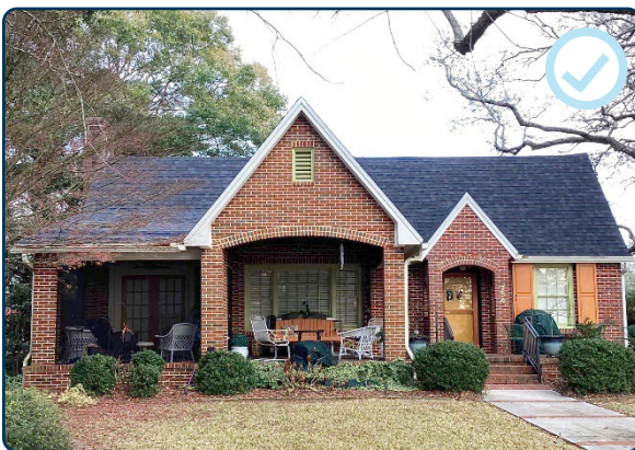
Figure 68: Appropriately maintained brick masonry residence in the DeFuniak Springs Historic District.
