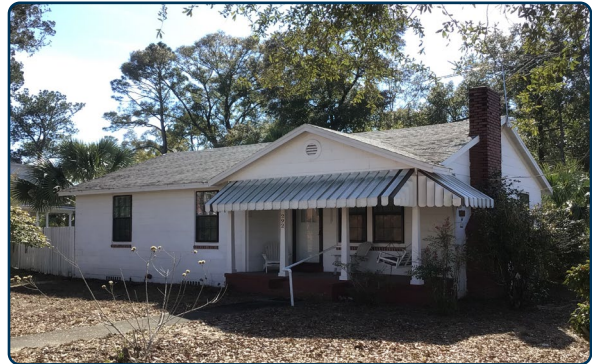
Figure 24: Above is an example of residential Masonry Vernacular style building in the DeFuniak Springs Historic District.
