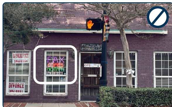
Figure 56: Not acceptable on the front façade of a commercial building.
