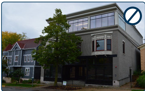
Figure 118: Inappropriate rooftop addition with incompatible fenestration.
