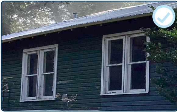
Figure 66: Appropriately preserved wood windows that need to be repainted to protect the wood.
