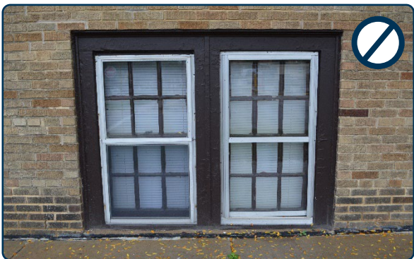
Figure 82: Inappropriate storm windows that obscure the original windows.
