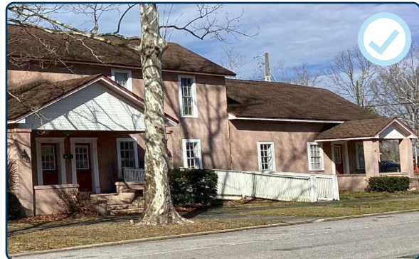
Figure 59: Appropriate ramp addition on the side elevation of a property in the commercial district.
