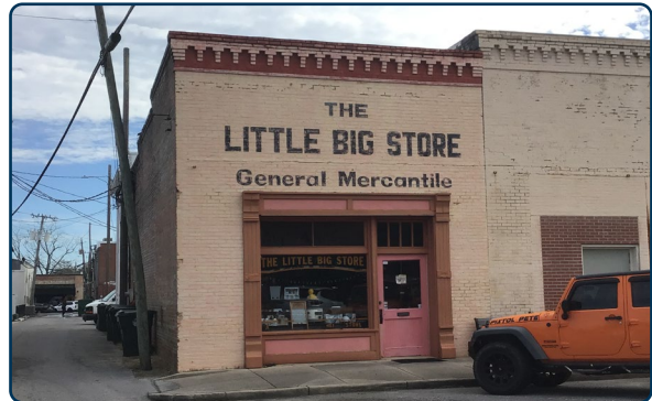
Figure 25: Most masonry vernacular style buildings in the DeFuniak Springs Historic District are commercial.
