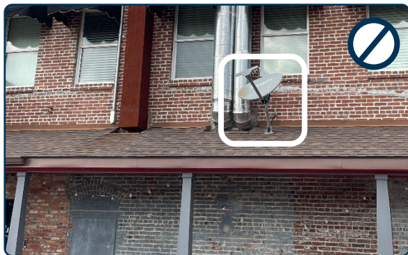
Figure 110: Inappropriate location of a satellite on the front façade of a commercial building.
