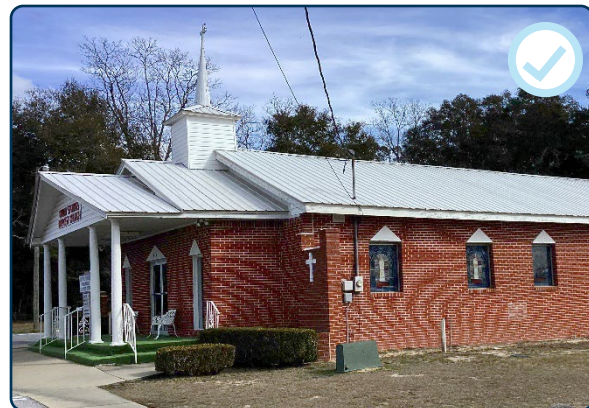
Figure 56: Both residences and religious buildings within the district feature brick masonry façades on wood frames.
