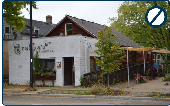
Figure 116: Inappropriate front commercial addition that obscures the historic residence.
