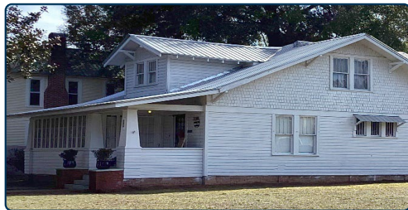
Figure 63: Historic residence that features multiple wood siding types.
