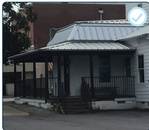
Figure 57: Simple metal ADA railing leading to the commercial property from an adjacent parking lot.
