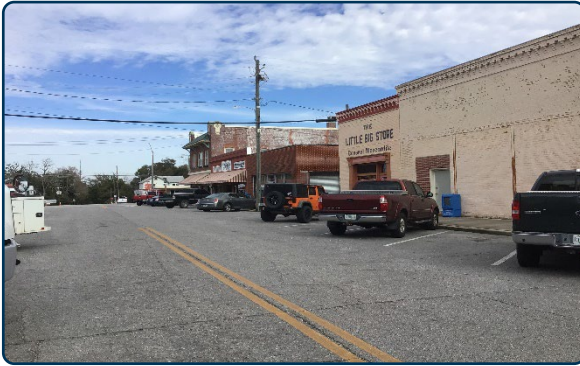
Figure 31: Example of a paved street within the commercial core of the district.
