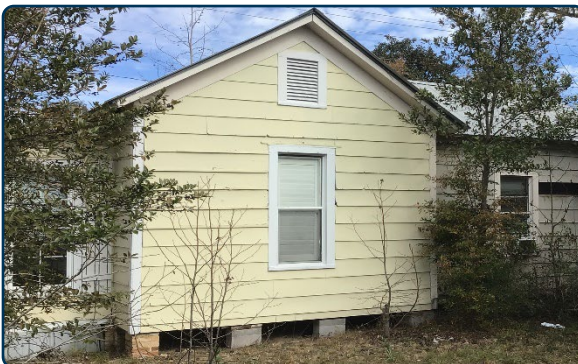
Figure 74: Example of a typical brick/concrete block pier foundation.
