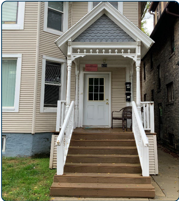
Figure 130: Porch flooring and steps replaced with compatible substitute material similar in visual qualities.
