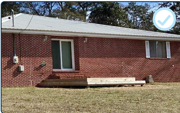
Figure 80: Appropriate deck addition on the rear of a residence that just needs painted to protect the wood.
