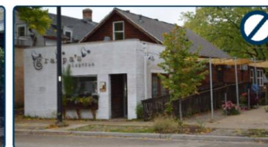
Figure 100: Inappropriate front commercial addition that obscures the historic residence.
