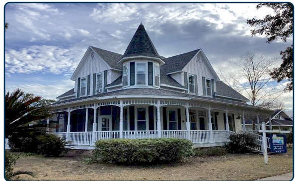
Figure 28: Above are examples of Queen Anne style buildings in the DeFuniak Springs Historic District.
