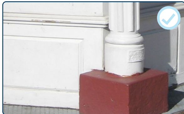
Figure 97: Appropriate replacement of a wood bulkhead on a historic storefront.
