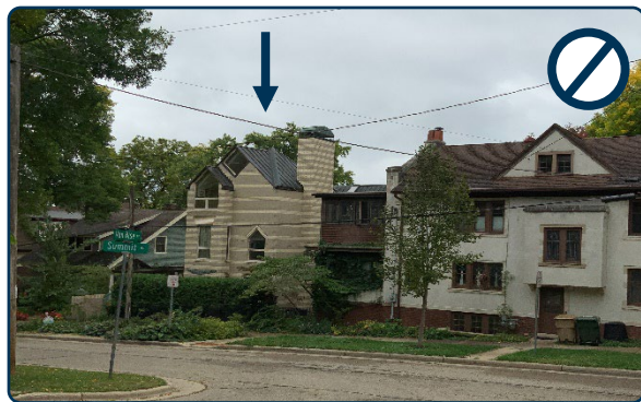
Figure 116: Inappropriate new construction with incompatible massing, materials, scale, height, and rhythm.
