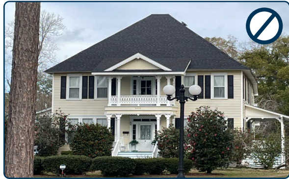
Figure 87: Inappropriate new roofing material and new roof shape on a historic residence that are not compatible with the residence's architectural style.
