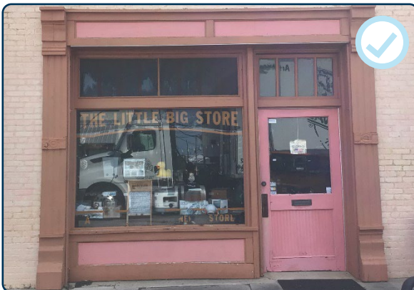
Figure 63: Historic commercial building that features wooden pilasters and ornamentation.
