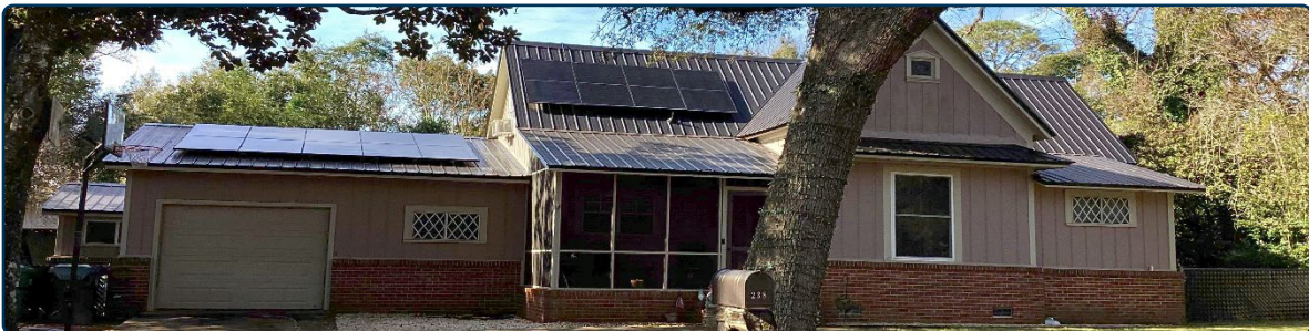
Figure 106: Example of solar panels appropriately installed on the roof of a historic residence.
