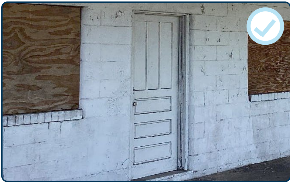
Figure 61: Appropriately preserved historic wood door.
