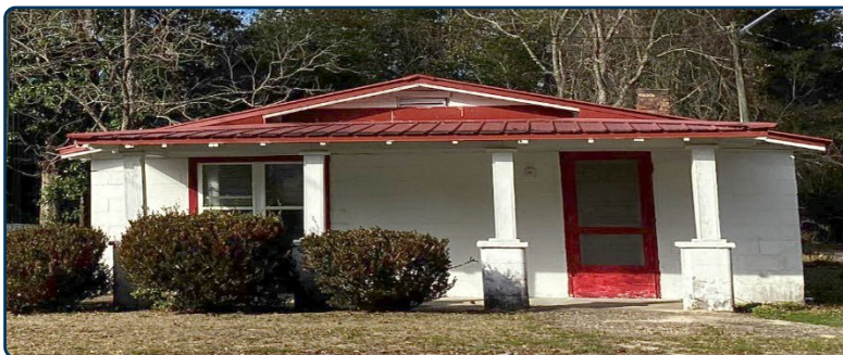
Figure 59: This historic building features exposed rafter ends and porch columns on masonry piers. The removal of these features would damage the integrity of the structure.
