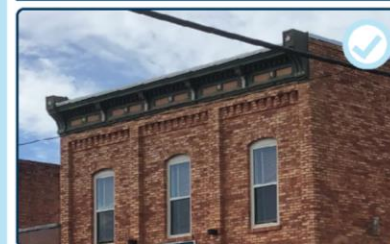
Figure 100: Preserved upper façade that features a pressed tin cornice on a two-story commercial building.
