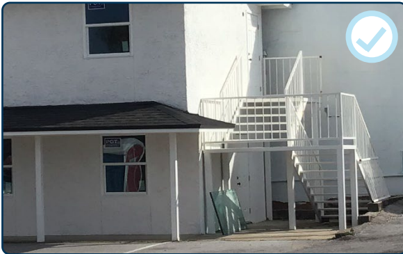
Figure 60: Compatible simple painted metal exterior stair on the side elevation of a commercial property.
