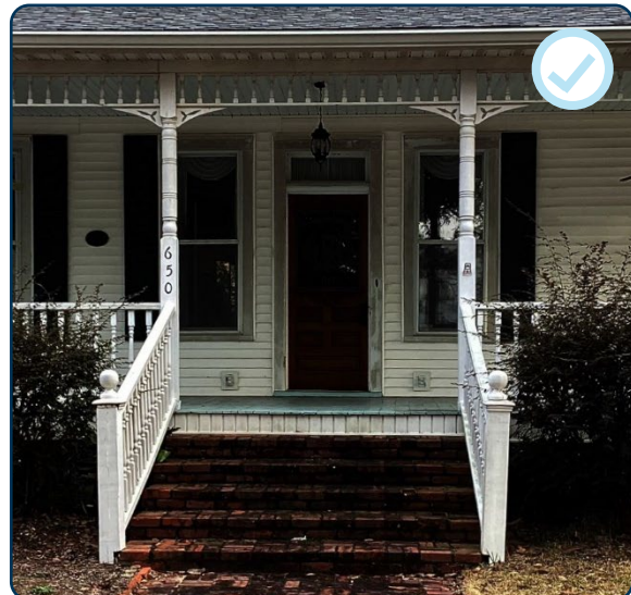
Figure 55: Appropriate railing on the front façade of a historic residence with a compatible design to the porch.
