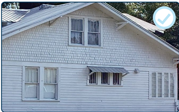
Figure 79: Appropriately preserved wood window types.
