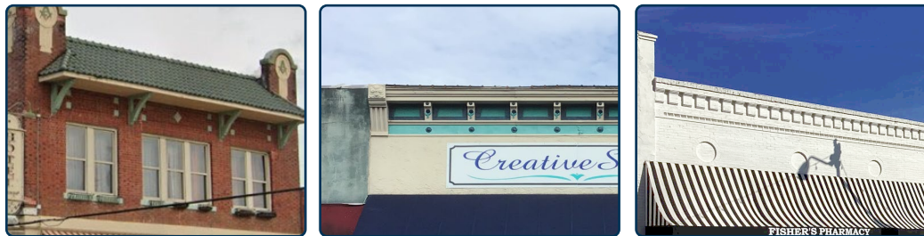
Figure 77: Examples of upper façades found on commercial buildings within DeFuniak Springs.
