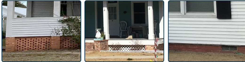
Figure 56: Examples of foundations found within DeFuniak Springs.
