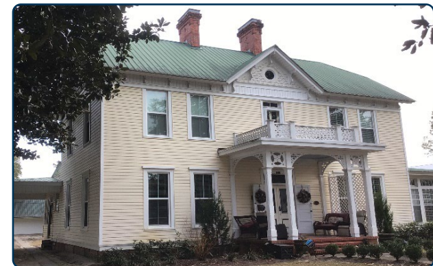
Figure 15: Example of a residential Double Pile building type in DeFuniak Springs.
